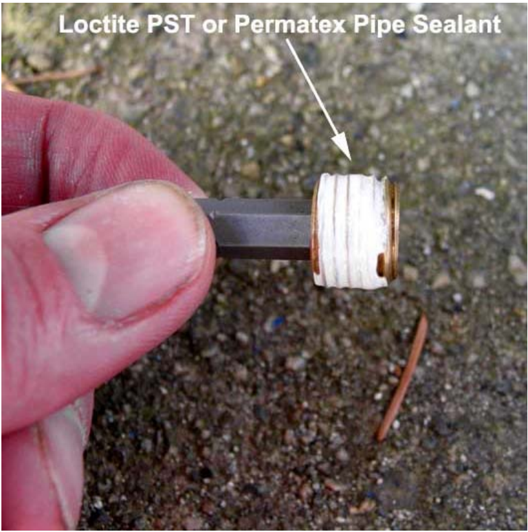
The plug prepared with sealant.
