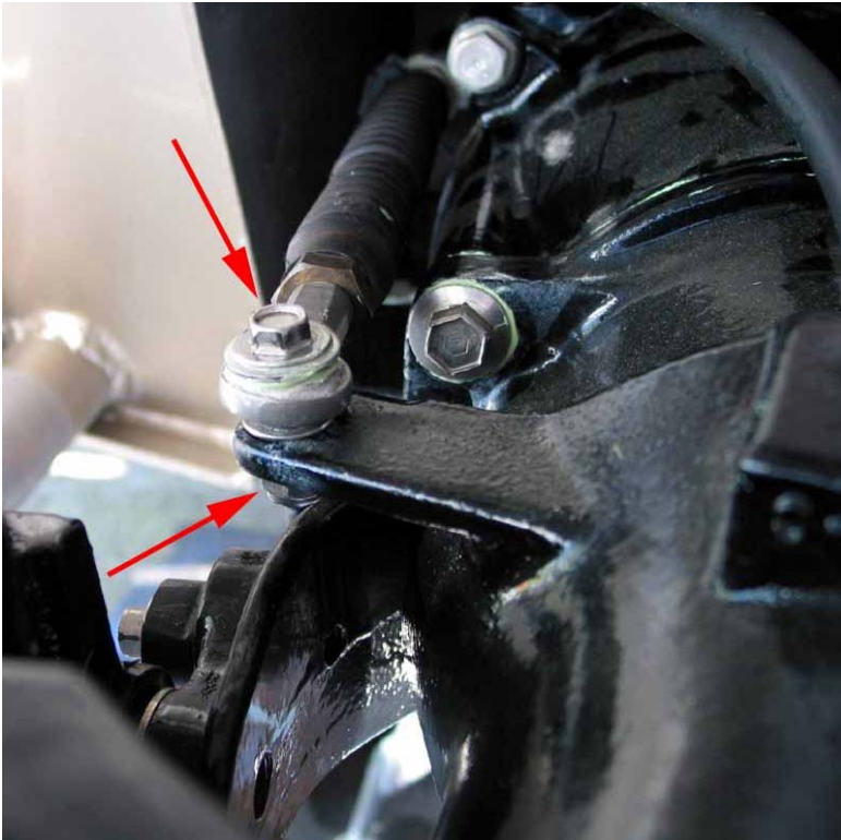
Picture 16: Removal of Steering Cable.
